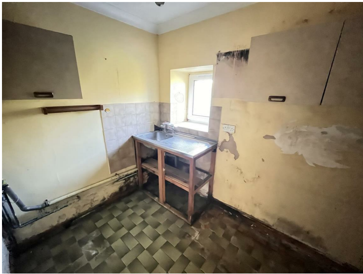
With stainless steel sink unit, plumbing for automatic washing machine
